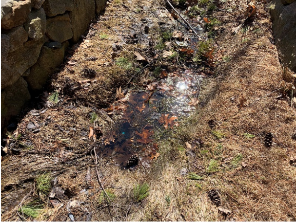
4 Brickyard Circle – 3 (Drainage Course)
