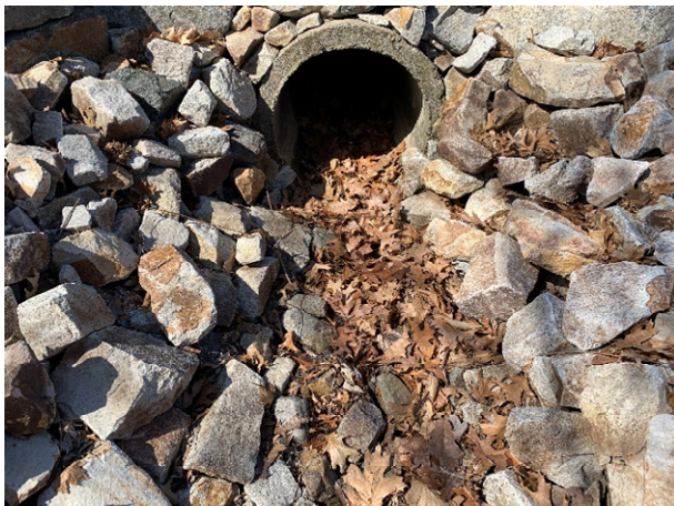
64 Gundalow - 1 (Drainage Course)
