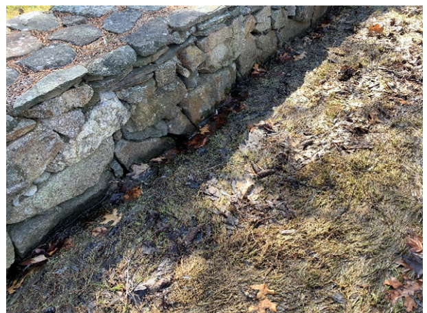
4 Brickyard Circle - 2 (Drainage Course)
