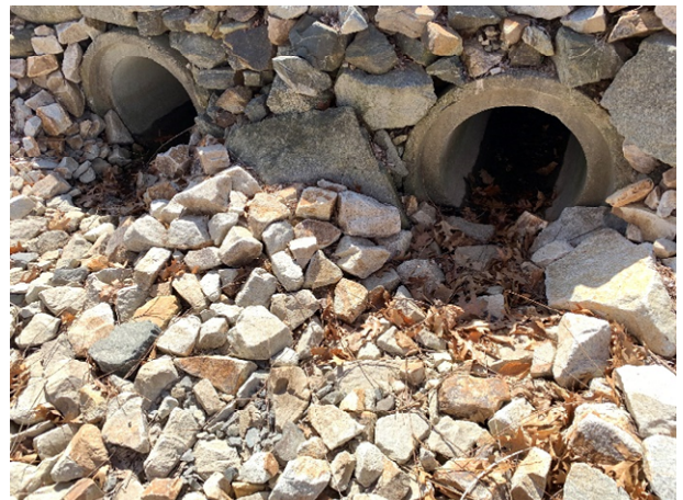
64 Gundalow - 2 (Drainage Course)
