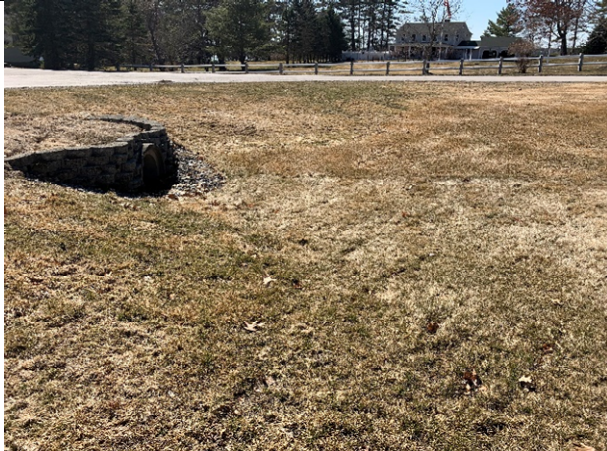
29 Gundalow - 1 (Drainage Area)
