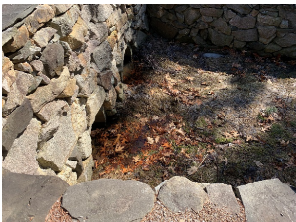
4 Brickyard Circle - 1 (Drainage Course)
